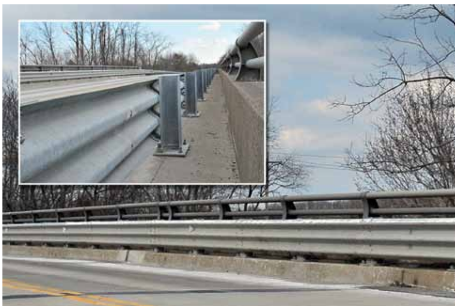
Figure 7-10. Delaware Thrie-Beam Retrofit
