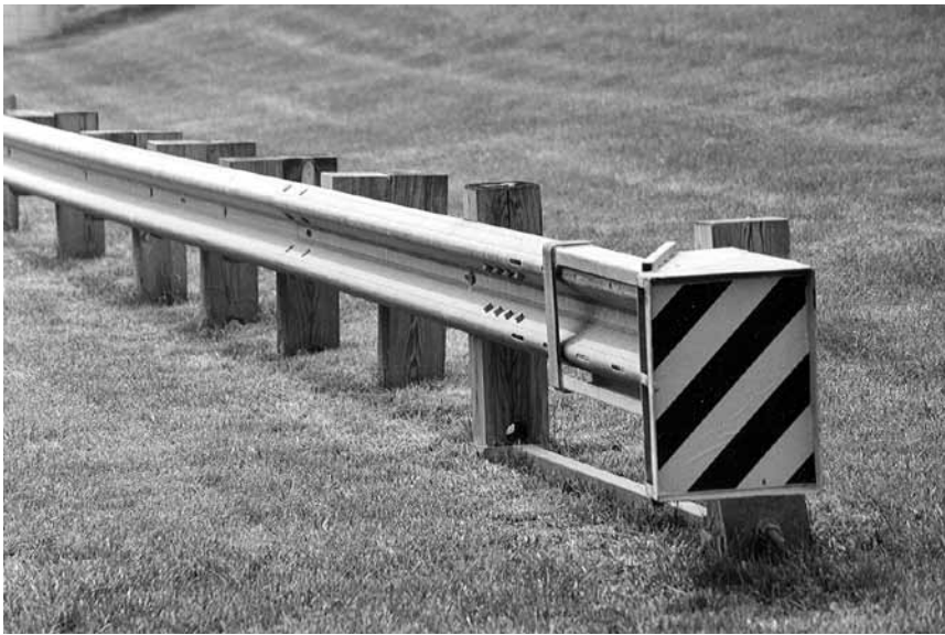
Figure 8-9. Flared Energy-Absorbing Terminal (FLEAT™)
