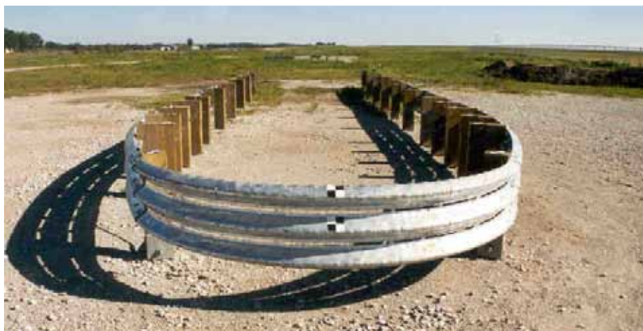
Figure 8-20. Bullnose Guardrail System
