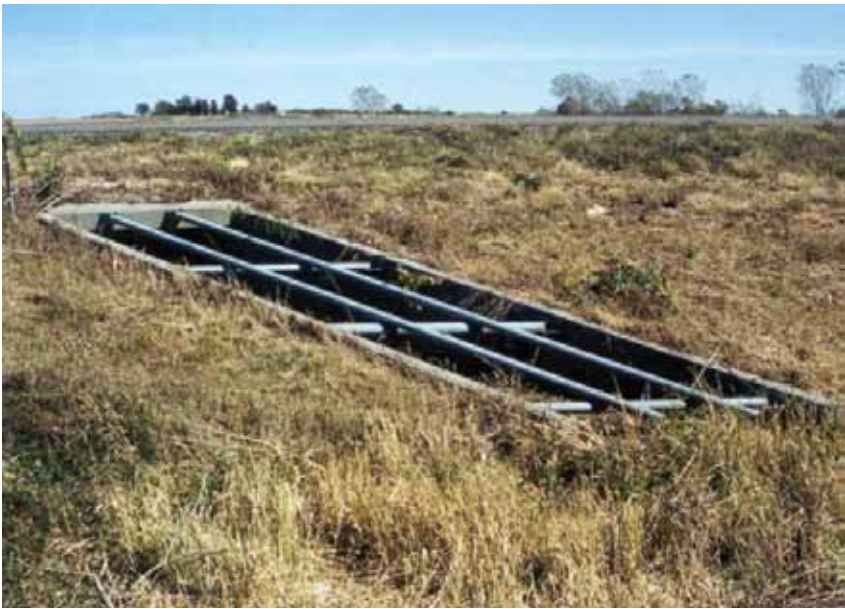
Figure 3-9. Safety Treatment for Cross-Drainage Culvert
