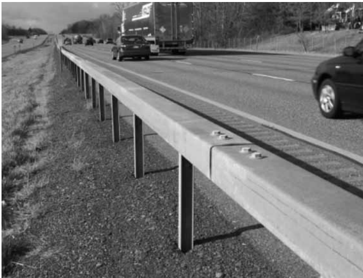
Figure 6-9. Box-Beam Median Barrier
