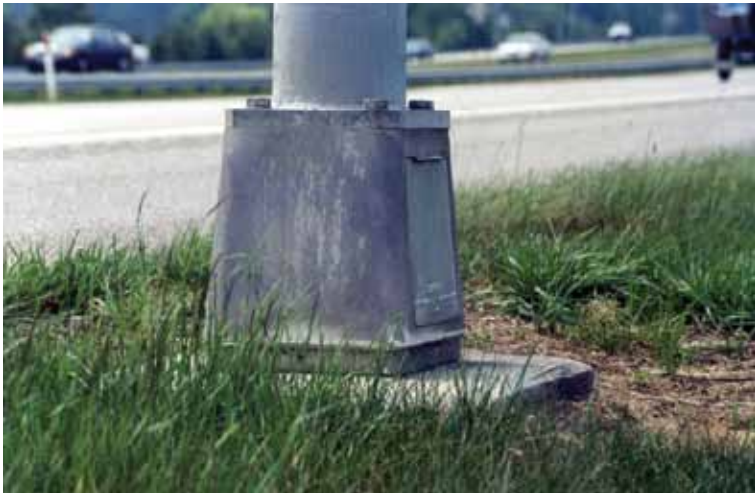
Figure 4-11. Example of a Cast Aluminum Frangible Luminaire
