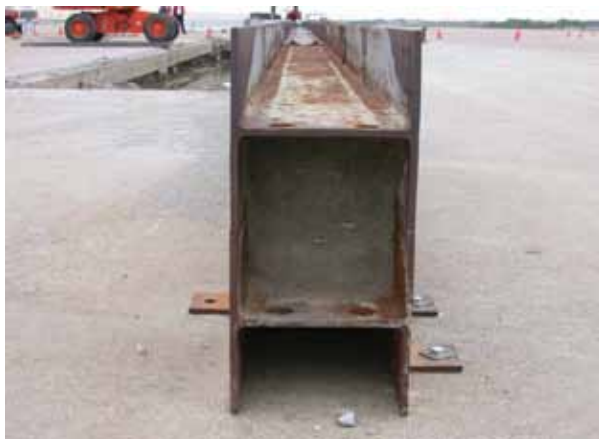
Figure 9-12. Iowa DOT Tie-Down Steel H-Section Temporary Barrier
