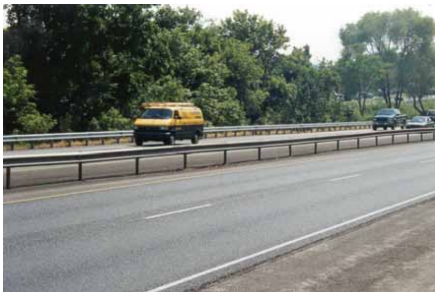
Figure 6-2. Weak-Post W-Beam Median Barrier
