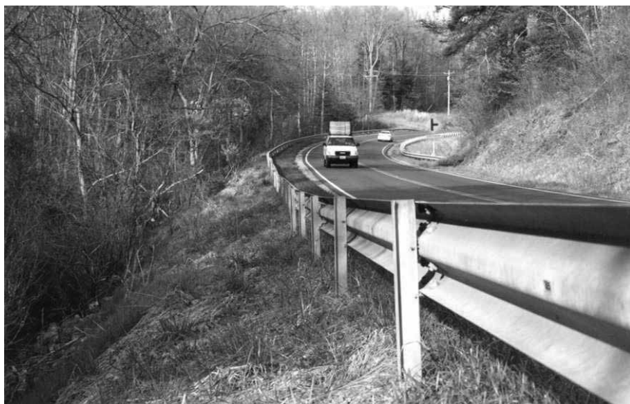
Figure 5-6. Weak-Post W-Beam Guardrail
