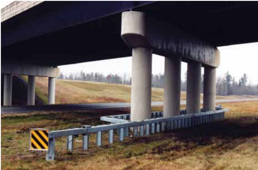
Figure 8-24. Bursting Energy Absorbing Terminal–Bridge Pier (BEAT-BP™) System
