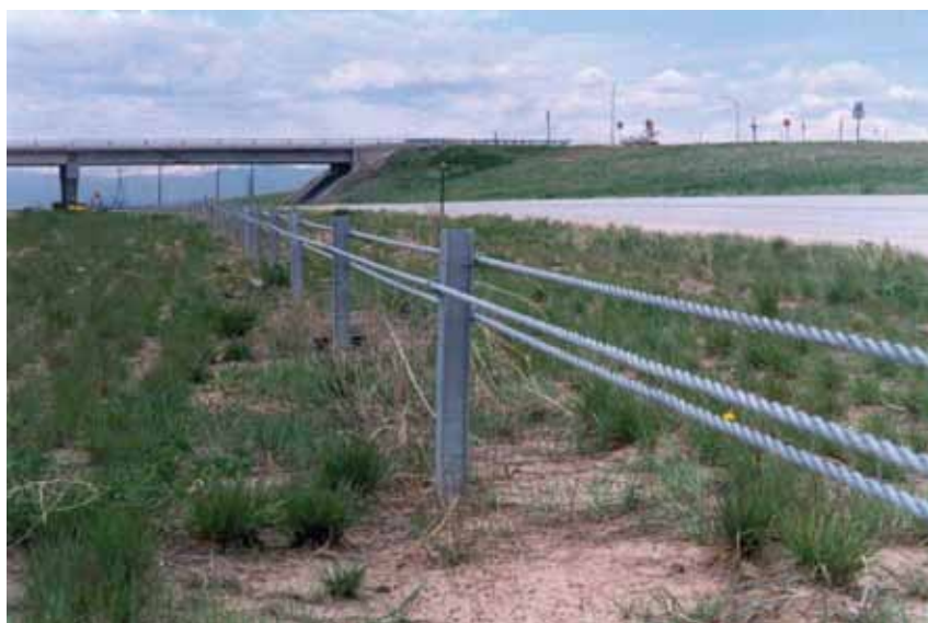
Figure 6-3. Three-Strand Cable Median Barrier
