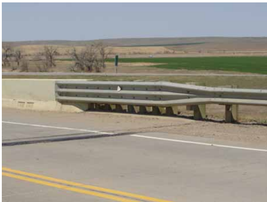
Figure 7-12. Thrie-Beam Transition to Modified Concrete Safety Shape
