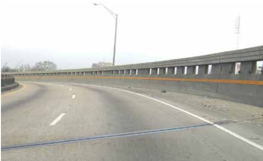
Figure 7-6. Texas Type TT Railing
