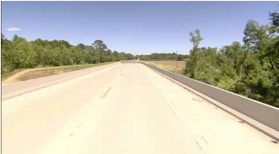
Figure 7-4. Concrete F-Shaped Bridge Railing
