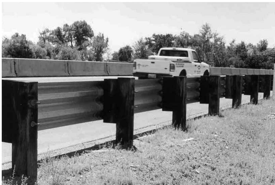
Figure 5-14. Wood-Post Thrie-Beam Guardrail
