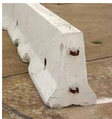
Figure 9-1. Iowa Temporary Concrete Barrier
