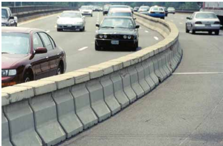
Figure 6-15. Standard Quickchange® Moveable Barrier System
