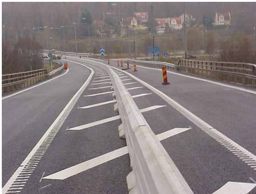
Figure 9-6. GPLINK® Pre-Cast Temporary Concrete Barrier
