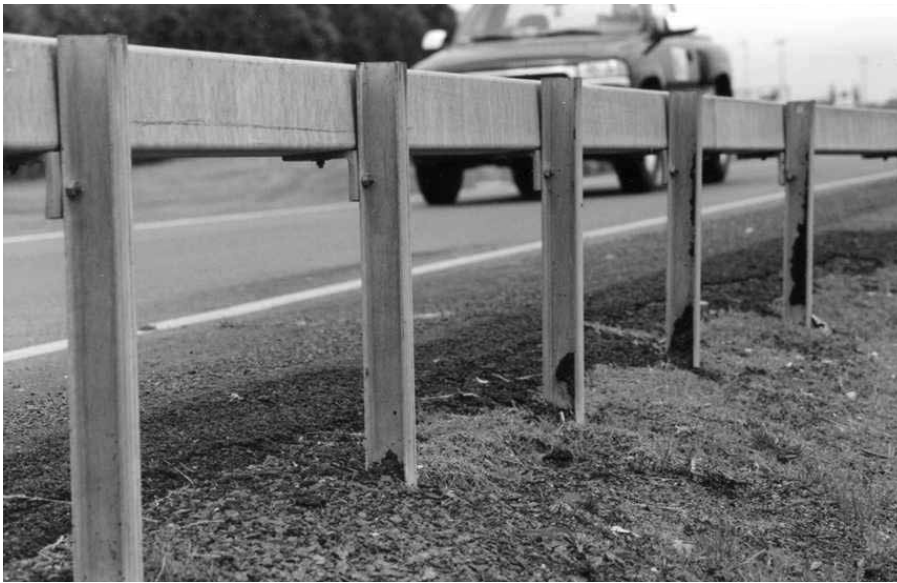
Figure 5-8. Weak-Post Box Beam Guardrail
