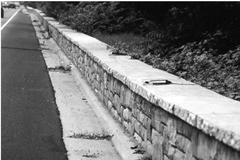
Figure 5-24. Precast Masonry Wall
