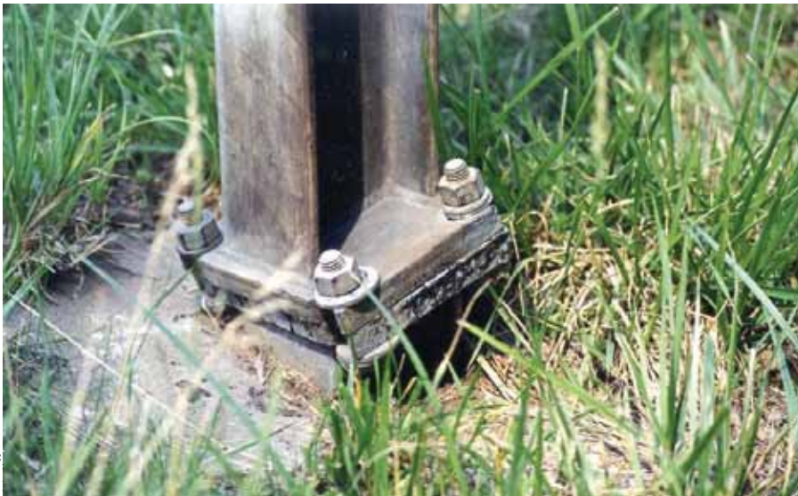
Figure 4-8. Unidirectional Slip Base for Small Signs
