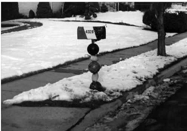
Figure 11-2. Examples of Hazardous Single Mailbox Installations
