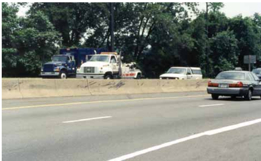
Figure 6-13. Concrete Safety-Shape Median Barrier
