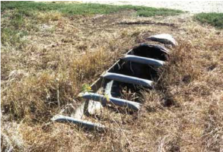
Figure 3-12. Safety Treatment for Parallel Drainage Pipe
