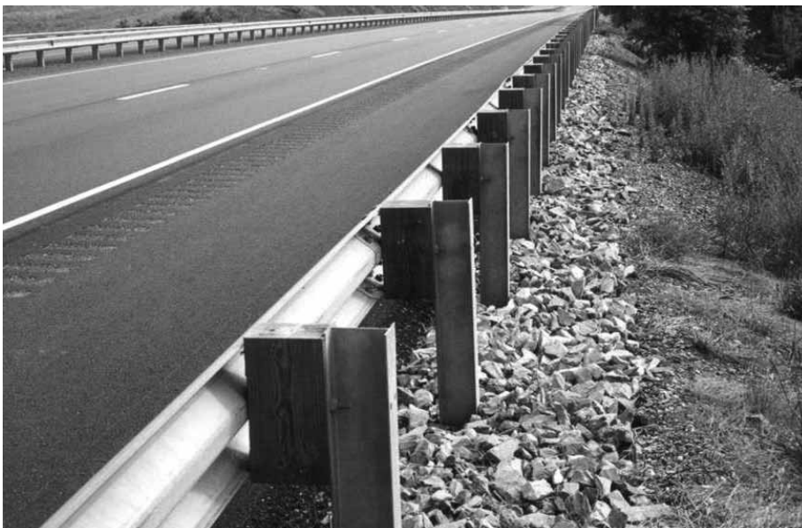
Figure 5-9. Steel-Post W-Beam Guardrail with Wood Blockouts
