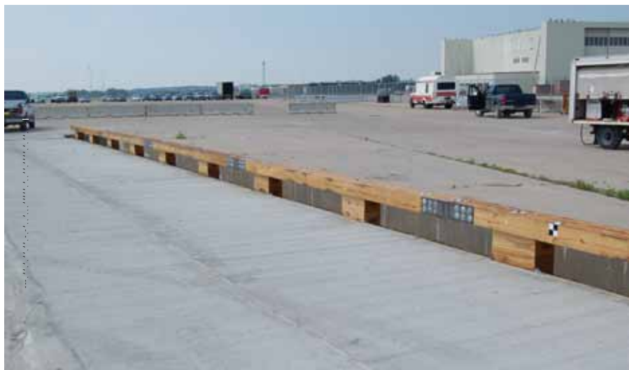
Figure 7-1. Curb Type Glu-Lam Timber Railing
