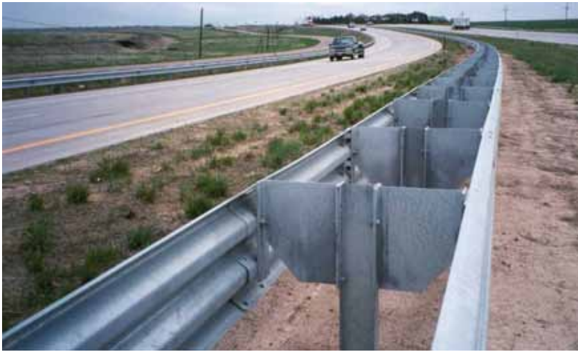
Figure 6-11. Modified Thrie-Beam Median Barrier
