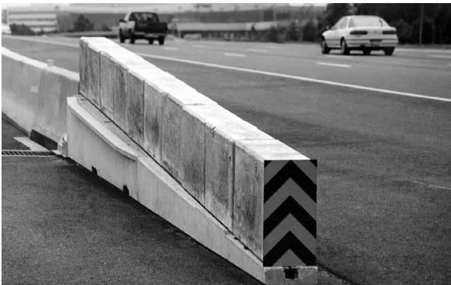
Figure 8-22. Advanced Dynamic Impact Extension Module (ADIEM™)
