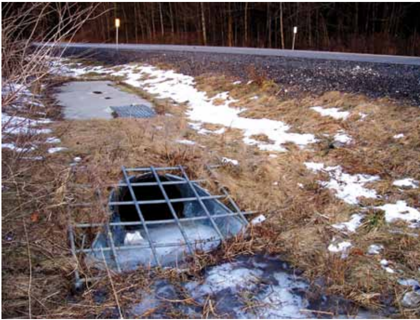
Figure 12-3. Reinforcing Steel Grate
