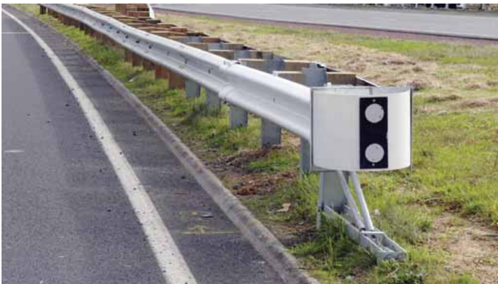
Figure 8-17. X-Tension™ Median Attenuator System (X-MAS)
