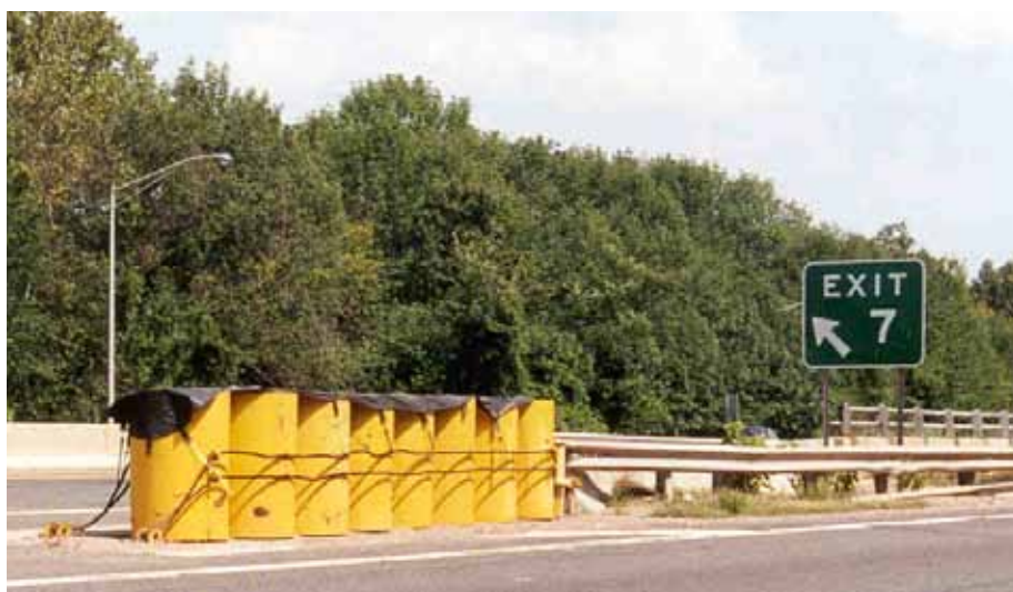
Figure 8-26. Narrow Connecticut Impact Attenuation System (NCIAS)
