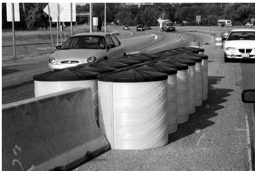
Figure 8-39. The Fitch Universal Barrel®
