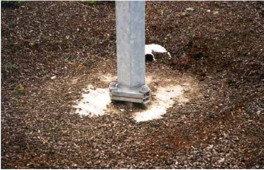
Figure 4-10. Oregon 3-Bolt Slip Base
