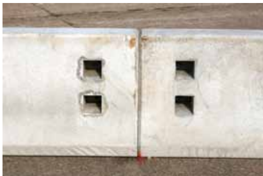
Figure 9-13. Quick-Bolt F-Shaped Concrete Safety Barrier
