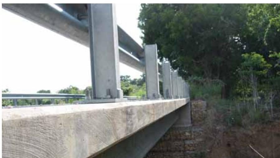
Figure 7-2. Texas T-6 Railing
