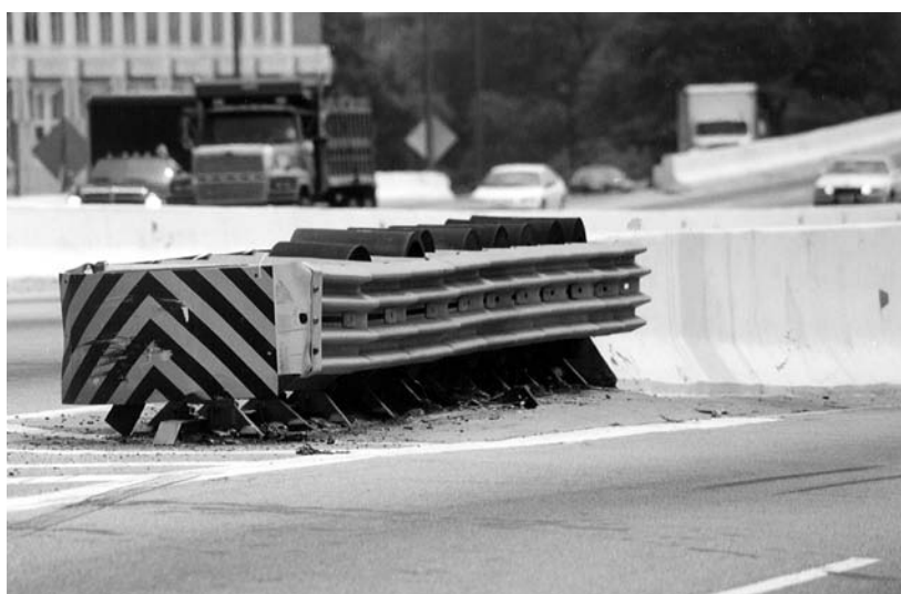
Figure 8-34. QuadGuard Elite
