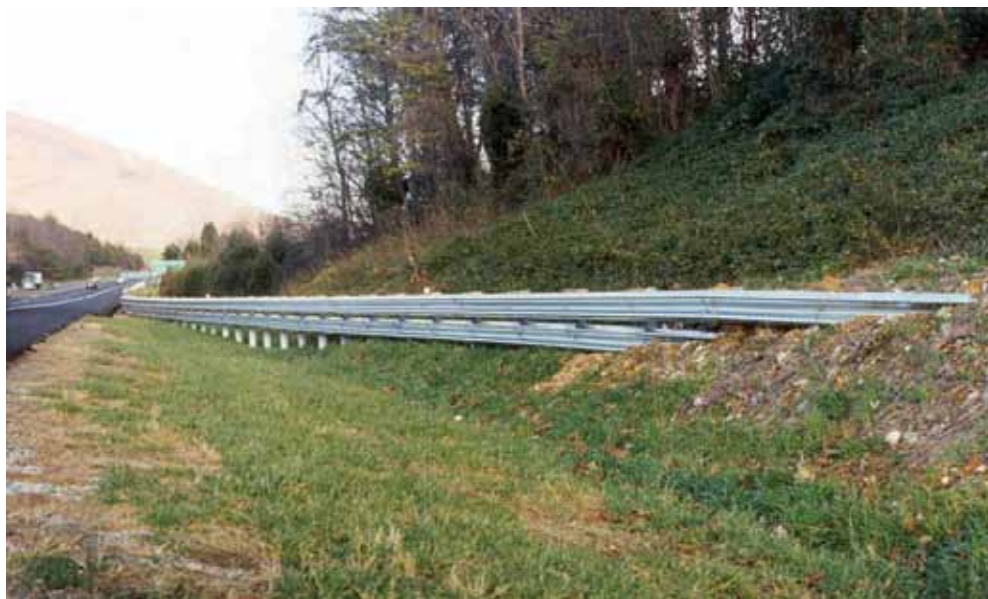
Figure 8-6. W-Beam Guardrail Anchored in Backslope
