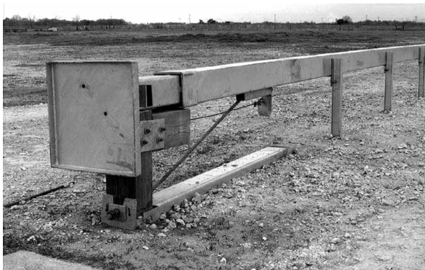
Figure 8-18. Wyoming Box-Beam End Terminal (WY-BET™)
