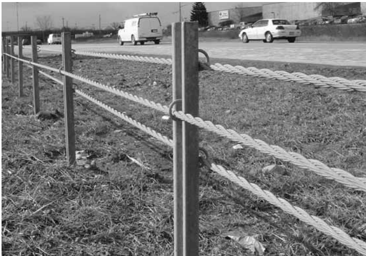
Figure 6-6. NU-CABLE™ High-Tension Cable System
