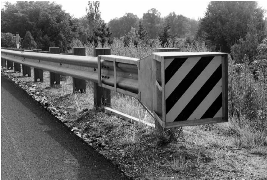
Figure 8-13. Sequential Kinking Terminal (SKT-350™)
