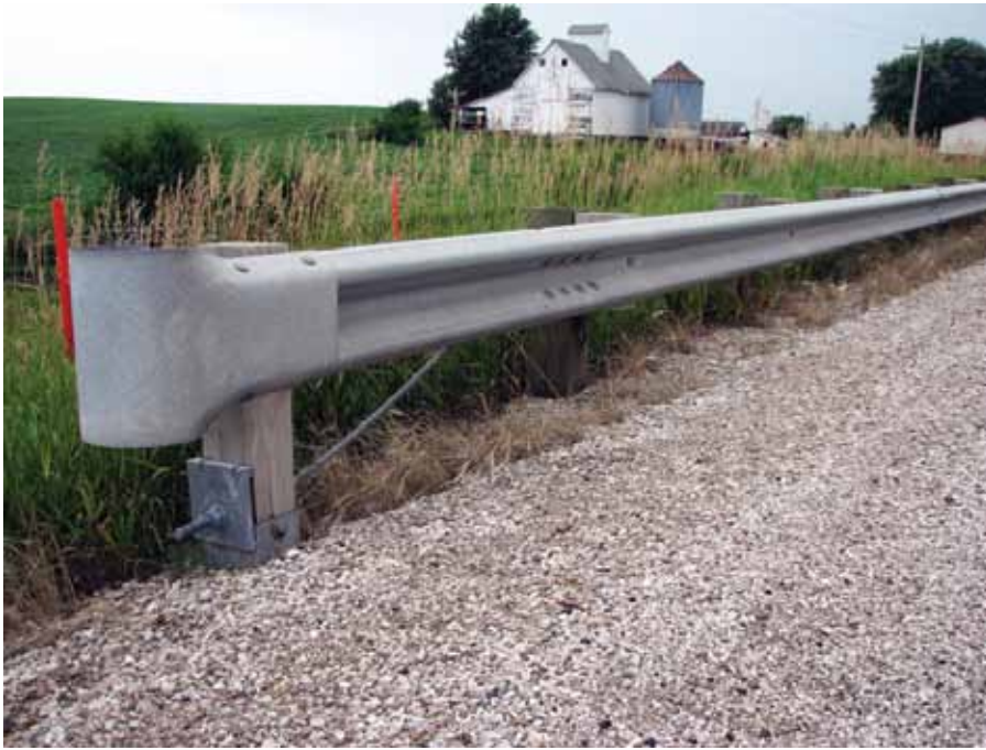
Figure 8-1. Trailing End W-Beam Guardrail Anchorage
