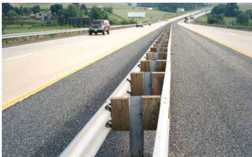
Figure 6-10. Strong-Post W-Beam Median Barrier
