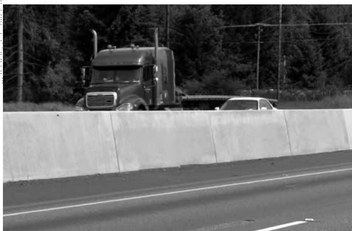
Figure 5-20. Constant Slope Barrier
