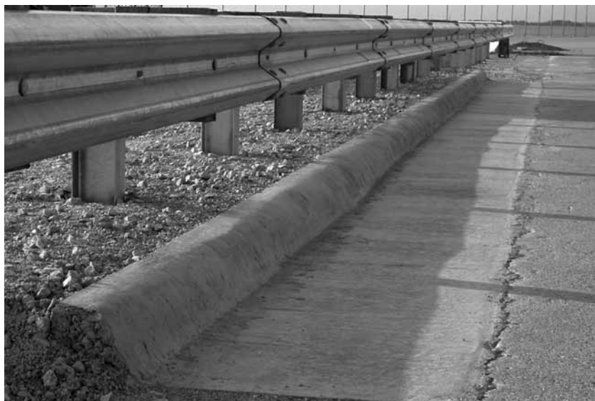
Figure 5-36. MGS Offset from Curb
