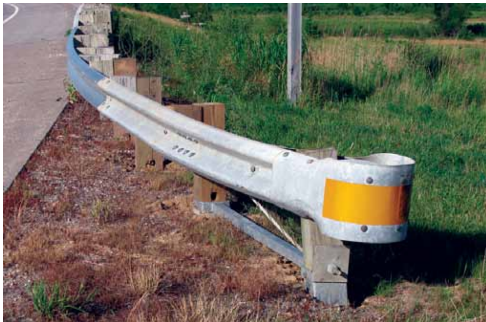
Figure 8-8. Modified Eccentric Loader Terminal (MELT)
