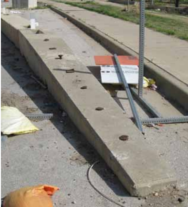
Figure 9-22. Slope-End Treatment for Low-Profile Portable Concrete Barrier
