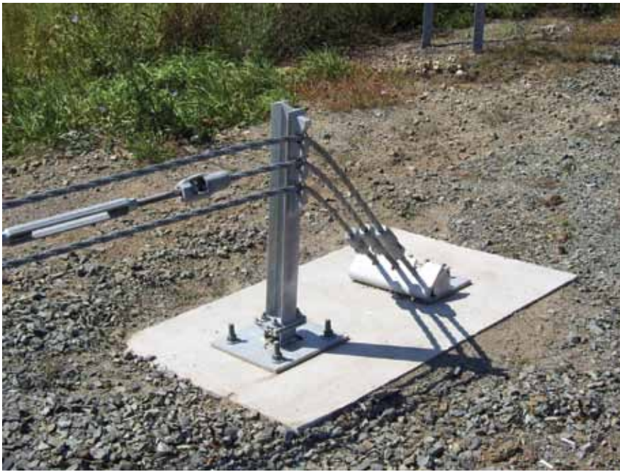
Figure 8-4. Three-Strand Cable Terminal
