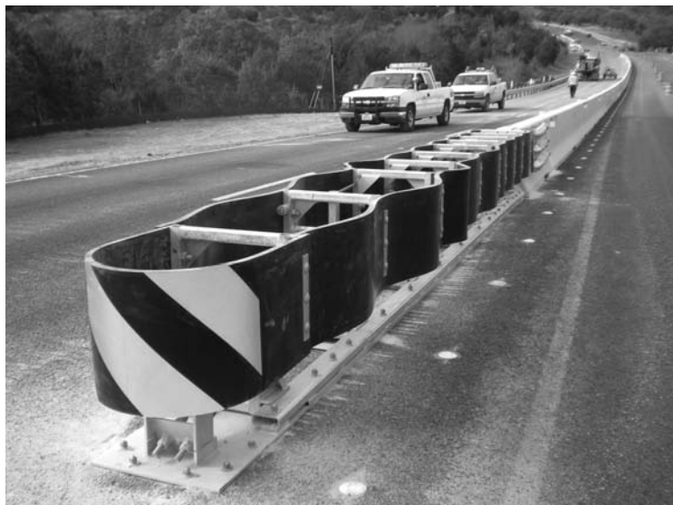
Figure 8-33. Hybrid Energy Absorbing Reusable Terminal (HEART™)
