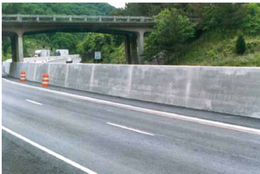
Figure 6-14. Single-Slope Concrete Median Barrier
