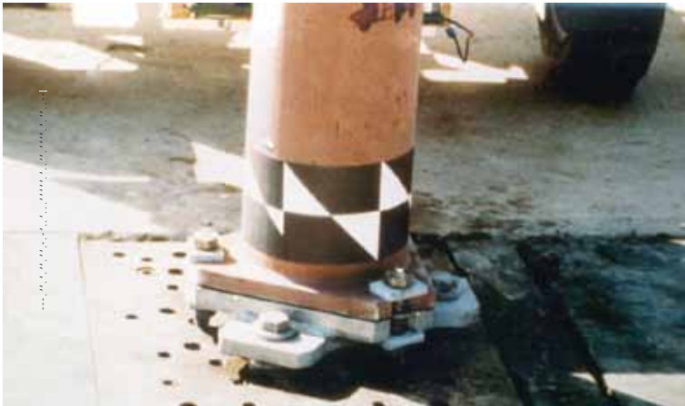
Figure 4-12. Example of a Luminaire Slip Base Design
