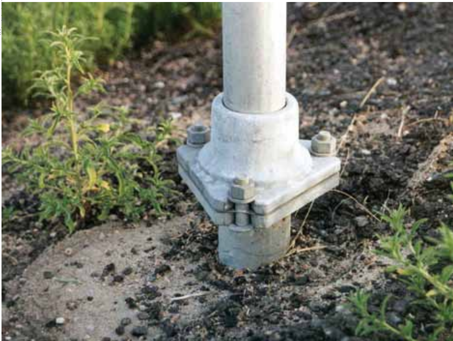
Figure 4-9. Multidirectional Slip Base for Small Signs
