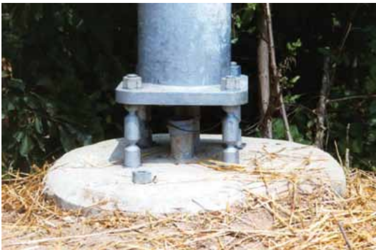
Figure 4-13. Example of a Frangible Coupling Design
